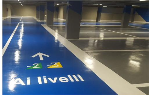
**Rivestimento autolivellante liscio (1,0 mm)**
